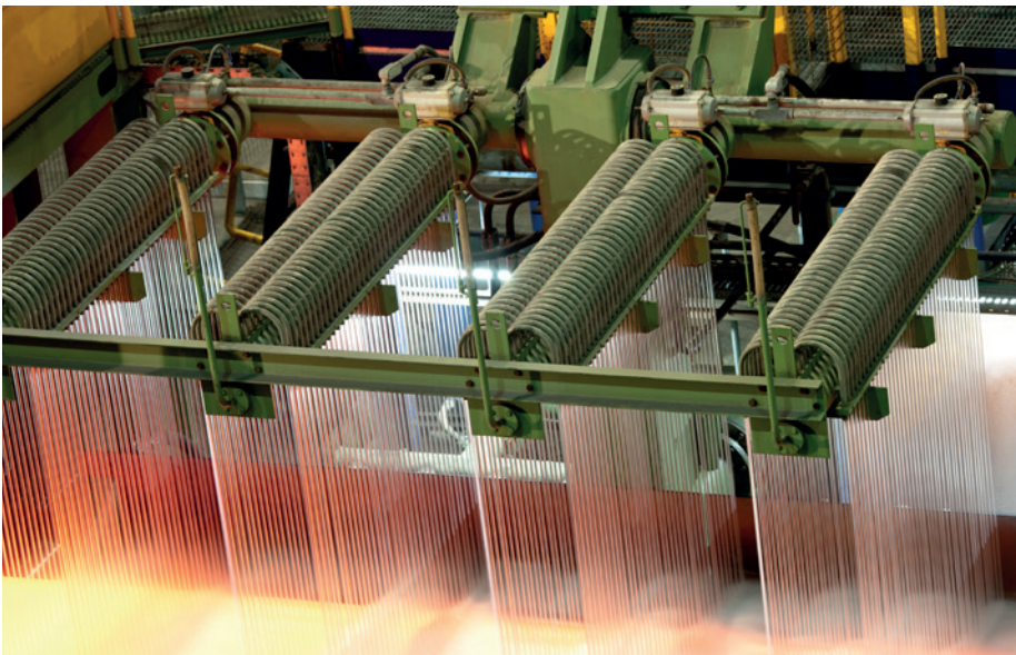
Cooling groups of the existing laminar cooling system (Picture: SMS group)
