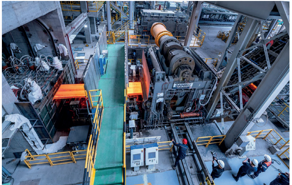
Discharge area of the thin slab casting machine at Yukun Iron & Steel (Photo: Danieli)
