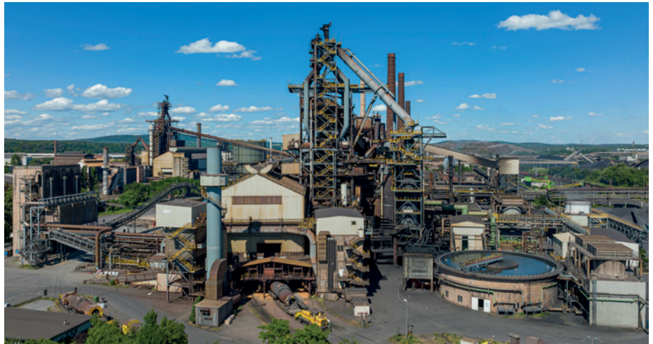
Blast furnace 4 at Rogesa will undergo a major upgrade this year (Photo: SMS group)
