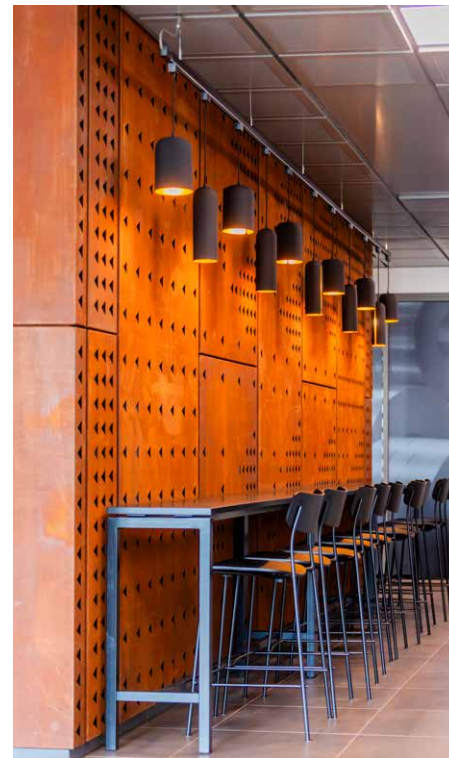
An artificial process was used to create a patina-like surface for this interior cladding (Photo: SSAB/Jaakko Mylly)
