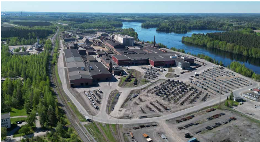
The Imatra steel complex will be connected to the local district heating network (Picture: Ovako)
