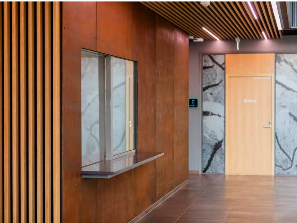
The front of the reception desk is made with ballistic protection Ramor 500 W steel (Photo: SSAB/Nick Tulinen)
