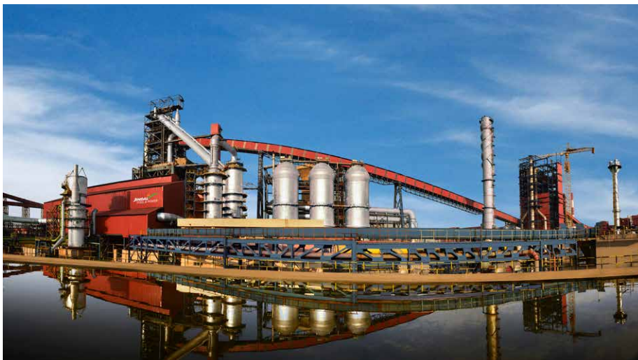
Blast furnace No. 1 at Jindal Steel and Power, Angul, India, will receive a new gas injection system (Photo: Primetals Technologies)
