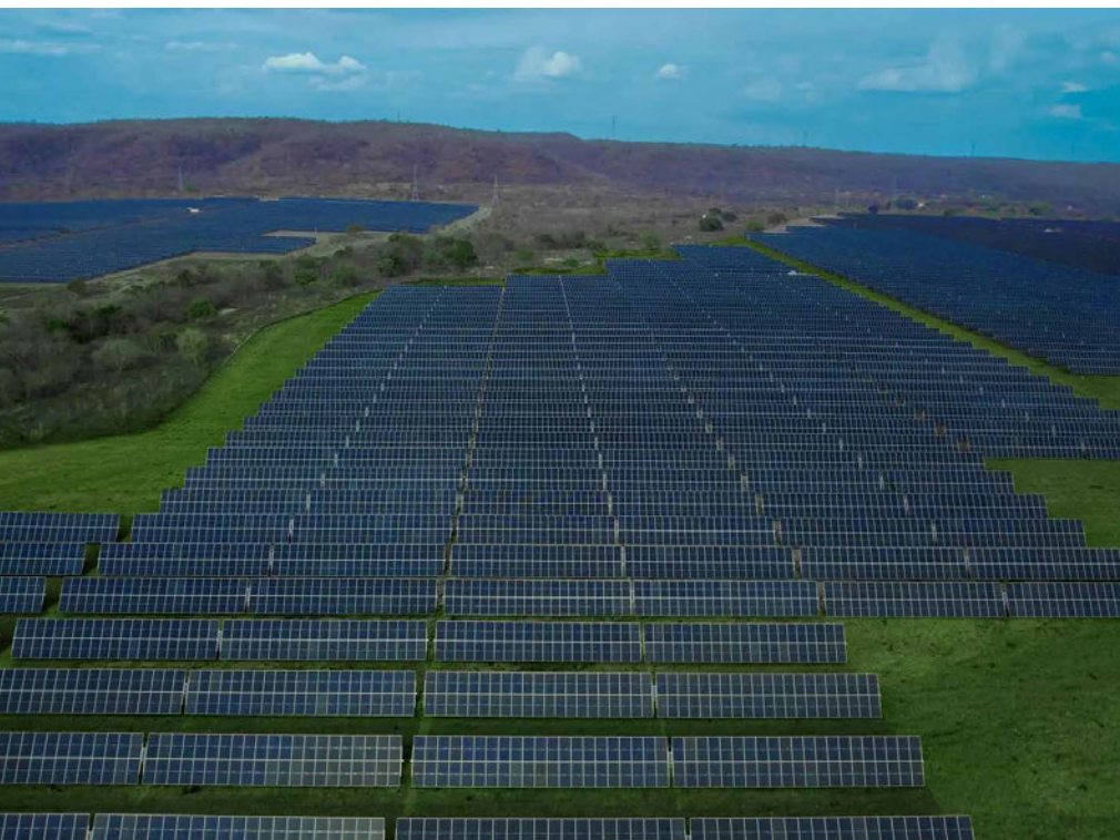
Construction of Luiz Carlos Solar Photovoltaic Complex began in 2024 (Photo: Atlas)
