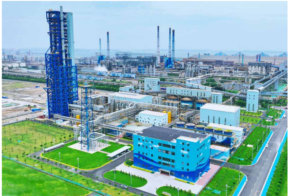
The DR plant at Baosteel Zhanjiang, China, achieved a production milestone during the performance test (Picture: Tenova)
